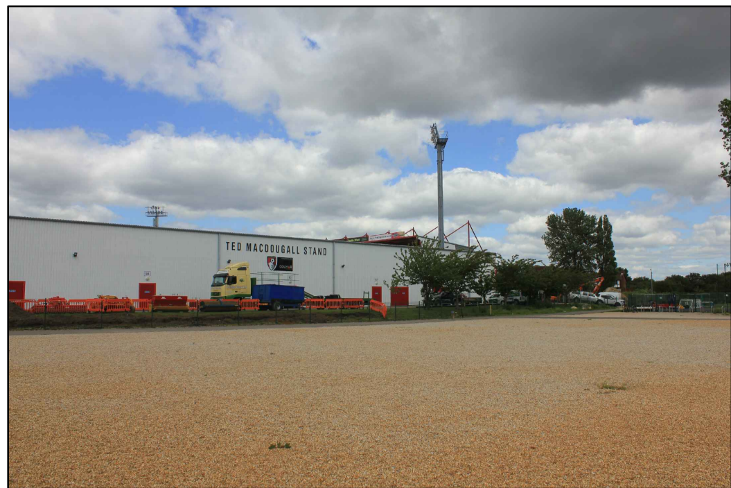
View looking North towards the South Stand
